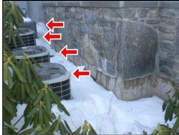
5.6 Picture 1 Air Compressors
