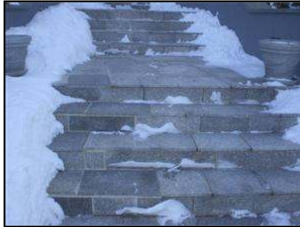
1.11 Picture 1 Front Walkway
