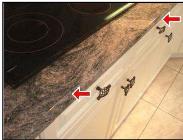
8.1 Picture 1 Loose Counter top
